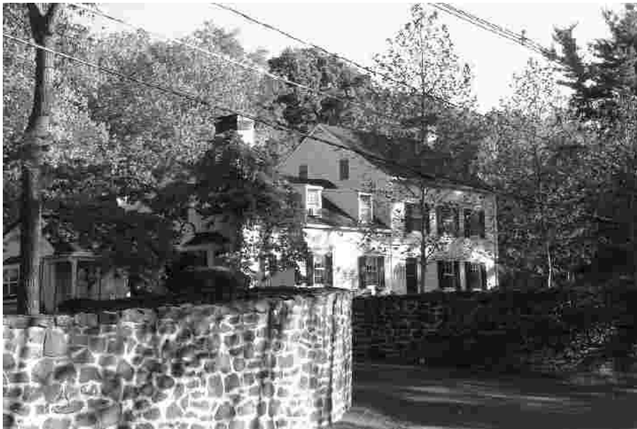
Pleasantville Road - Pleasantville Historic District (McCabe & Associates)
